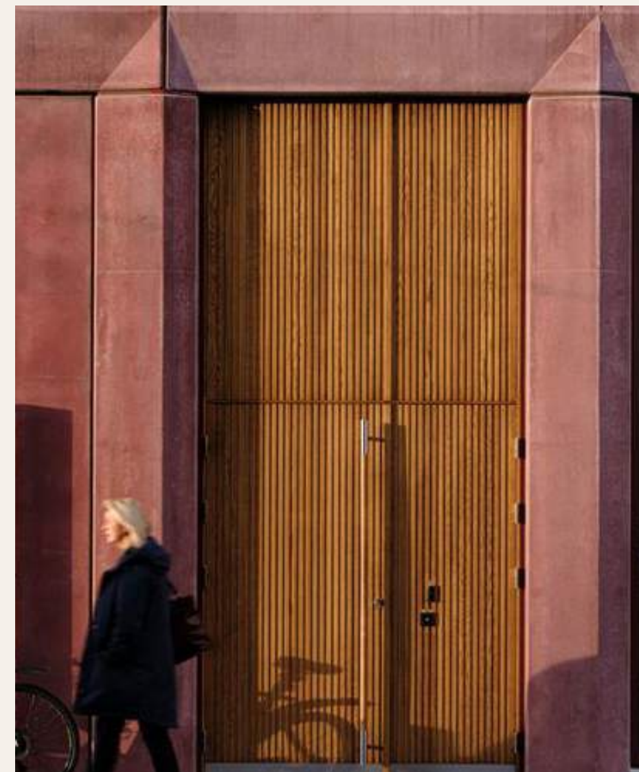
Example of the use of pigmented concrete and wooden framed door in main entrance.
